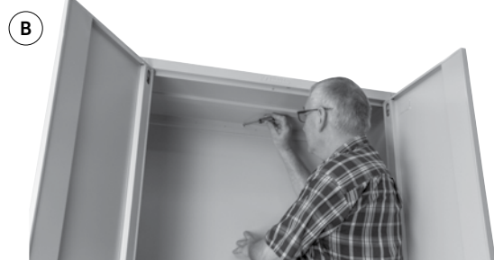
Fasten to the Back Panel with 3 x screws. Then, use a screwdriver to push the 'push-through' slots shown at 'A' into the Front Panel.
